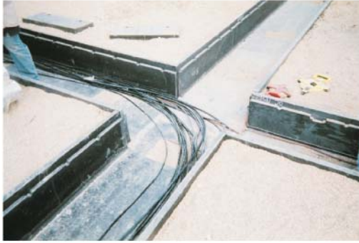
Gambar 10. Surface ducting
