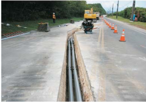
Gambar 11. Duct trenching
